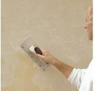
When the filler coat is thoroughly dry, a full surface trowel application of ArteTwin Effect Gold or Silver is possible.
