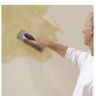
Subsequently the spots are blended to obtain a homogeneous surface. Trowel application has to be effected without emitting any scratching noises, the trowel should float softly on the surface.
